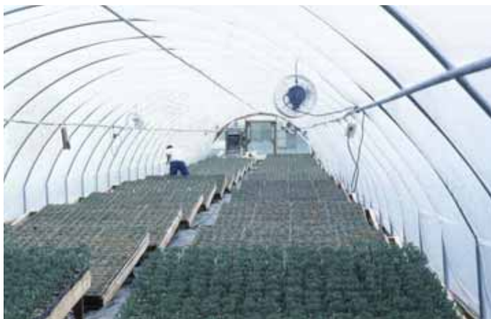
Photo 2. Greenhouse built to the slope. Stair-step beds keep plants growing on a level surface.
