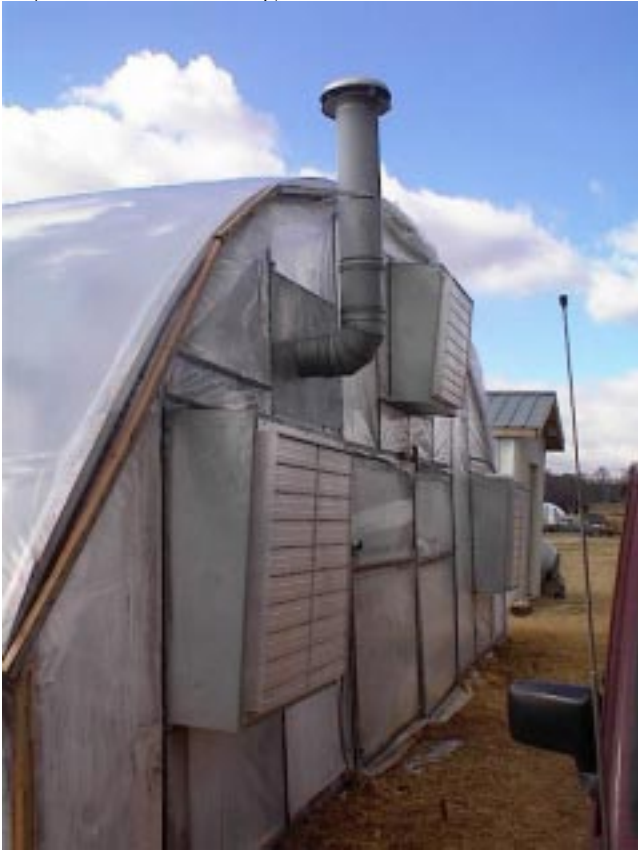
Vented heater exhaust stack
