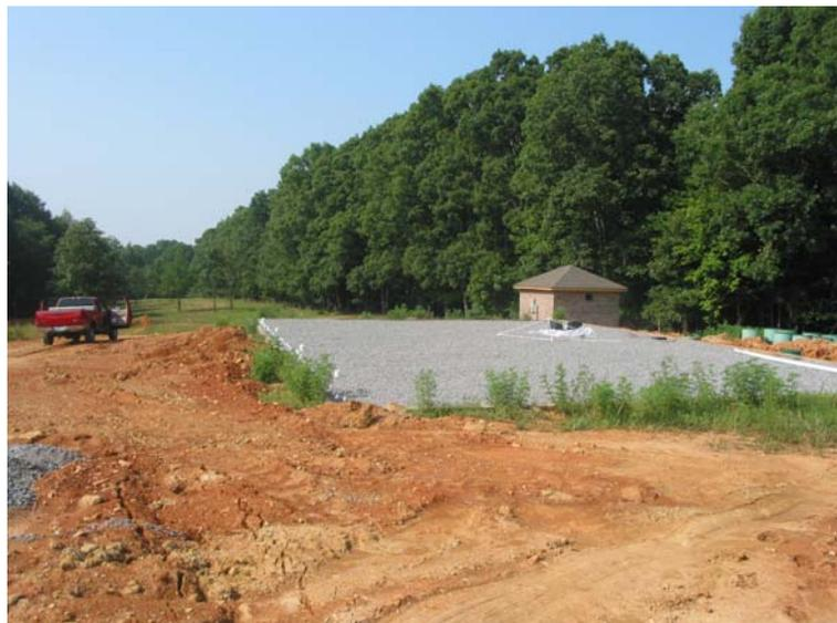
A recirculating sand filter and subsurface drip field. The drip field is in the background. This wastewater treatment system can handle 20,000 gallons per day.
